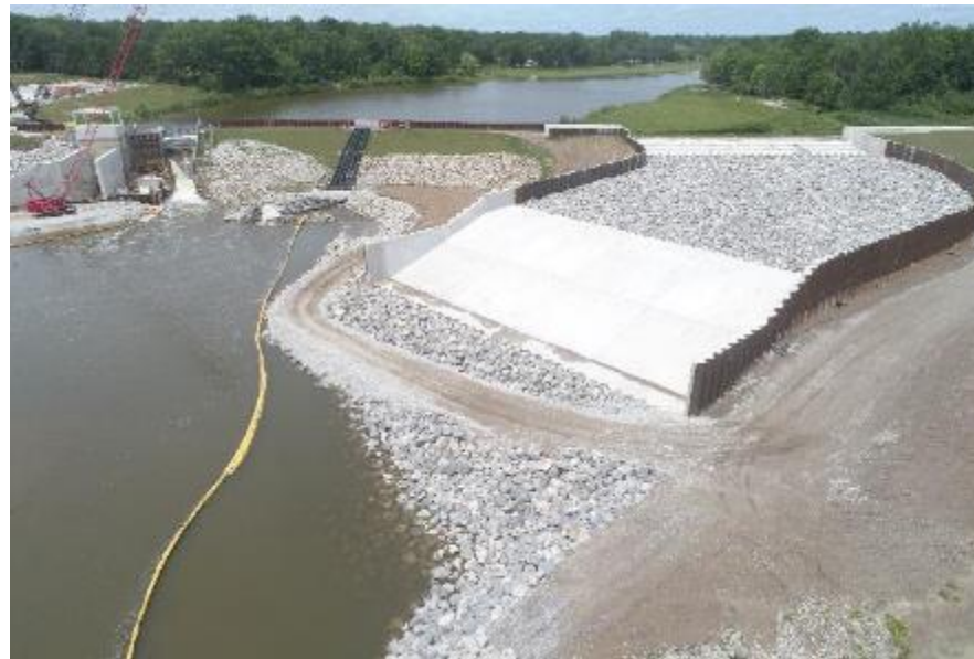
Auxiliary spillway, Siphon System and Left Embankment
