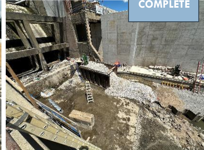
Downstream of Primary Spillway
