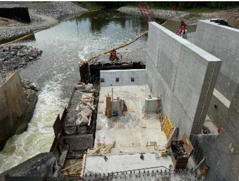
Downstream of Primary Spillway Bay No. 1
