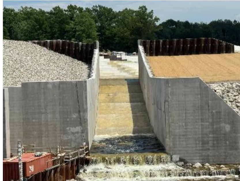
Auxiliary Spillway Chute
