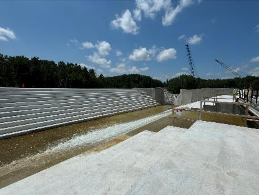
Auxiliary Spillway Basin
