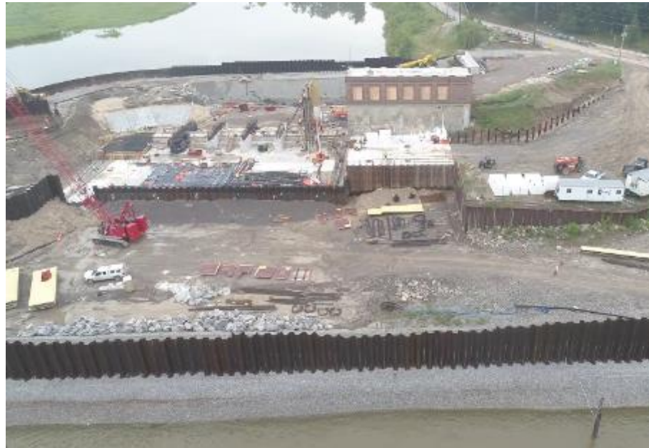
General site condition
