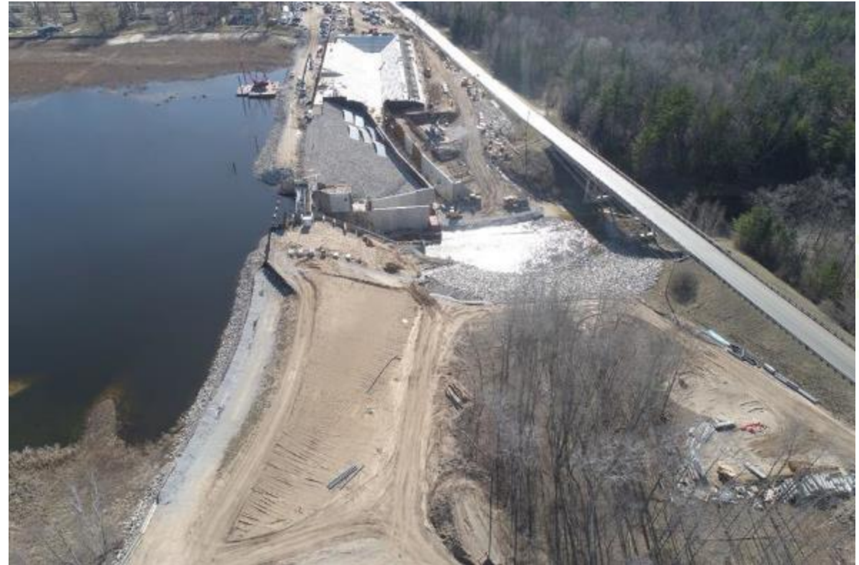
Secord Dam – Looking East
