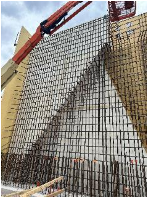
Pier No. 1 Formwork and Rebar
