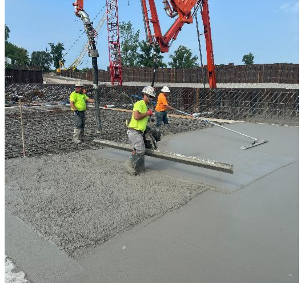
Pictured: Edging and finishing concrete apron slab on Sanford
